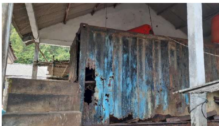
Figure 11. Broken ice factory.
